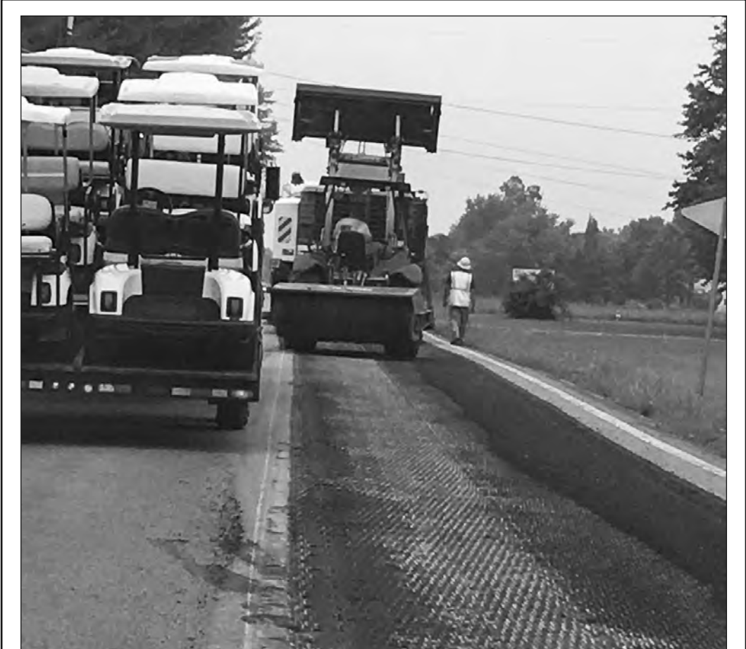
PHOTO BY ALLISON EVANS, THE PRESS A contractor for the Kentucky Transportation Cabinet is milling the existing U.S. 641 this week, taking up layers of asphalt for new pavement to be put down this month along the entire length of the road in Crittenden County.
